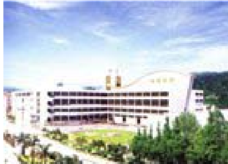
Facility II, Guangzhou, China
